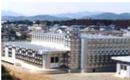
Water Storage Tank
